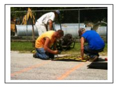
7. Continue to attach each adjoining section until crossing the roadway to the desired width. Before installing the final Safety Rider section, be sure your last end cap will fit into the last Safety main section. If not you should exchange that end cap for the proper end cap. Attach the other end cap using the same procedure.
